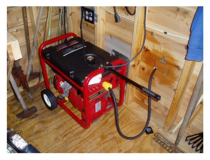
My Generator installation – inside a tool shed – exhaust is Vented outdoors
